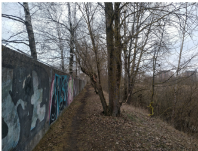
Figure 78. Existing concrete fencing and footpath (Photo: U. Valainis)
