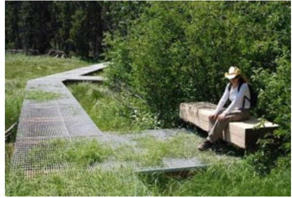
Figure 93. Example of a raised galvanised steel lattice walkway with seating benches
