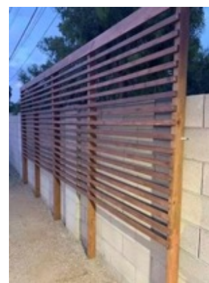
Figure 80. Concrete fencing wooden plank panels
